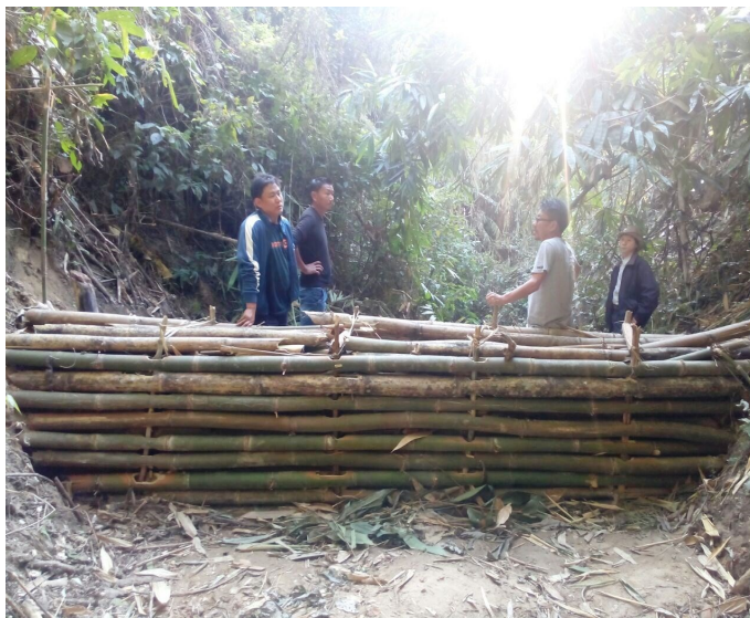
Bamboo based check dam in Zutovi Village
