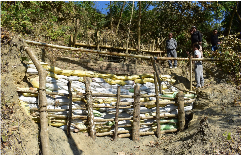
Sand filled bags Check Dams at Hovukhu Village
