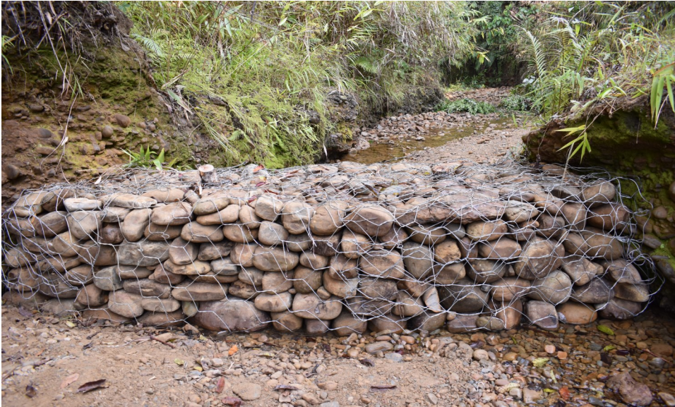
Gabion Structure at Ruzaphema village
